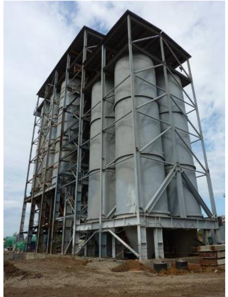
The steel structure of the Batch house
