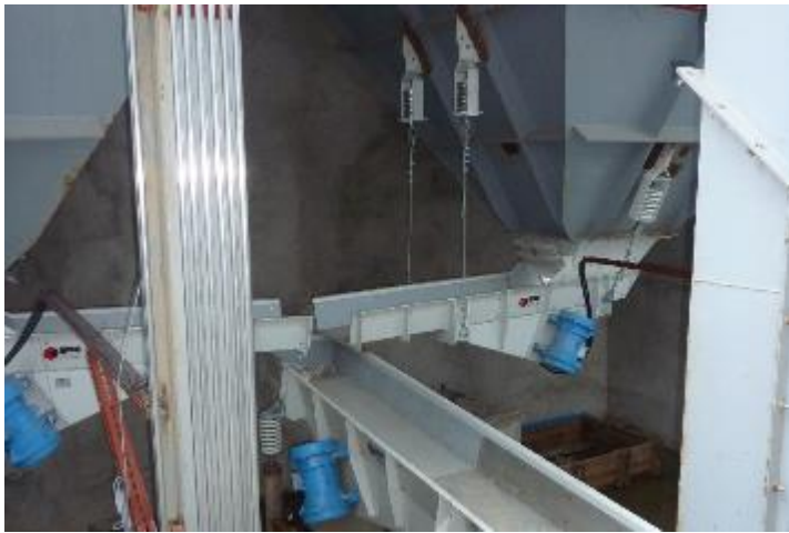
Hoppers beneath the rails - implementation
