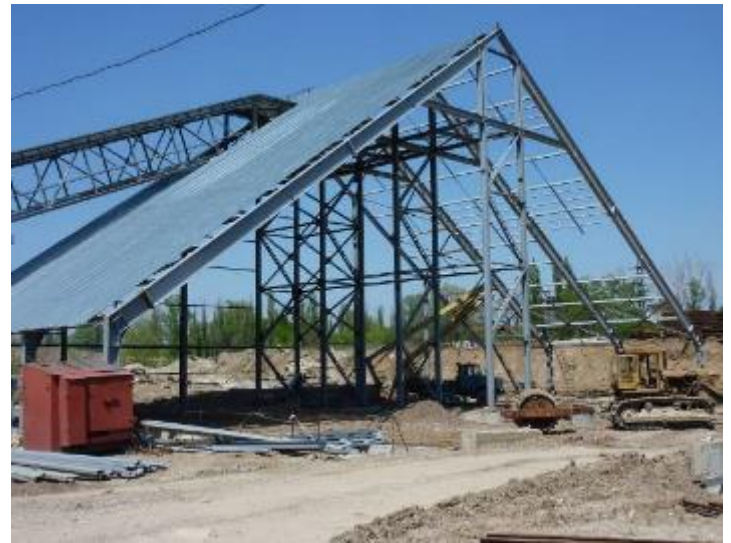
During the implementation of Sand storehouse
