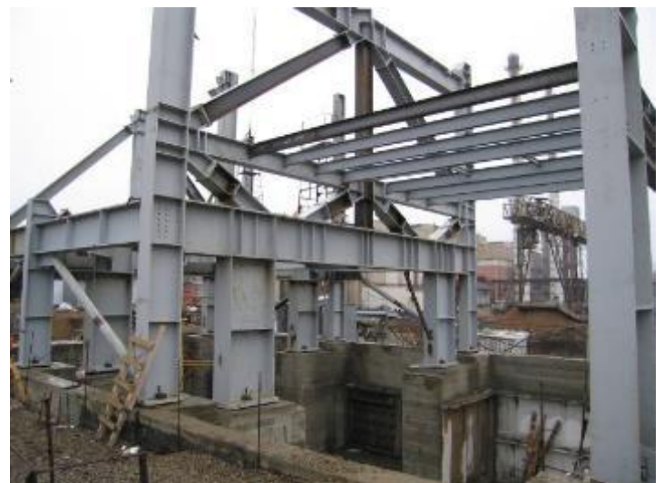
Fundamental construction of the Batch house – implementation
